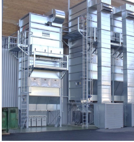
MultiStar jetfilter in de recyclingindustrie
